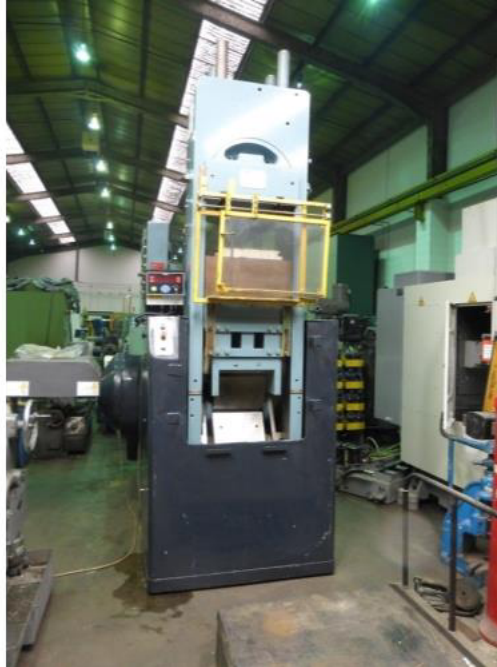
Photograph taken on site before machine has received any attention
